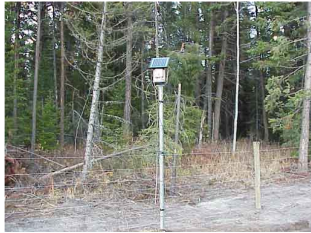
This set-up utilizes an energizer with a solar panel to provide a power source where electricity is not available.
