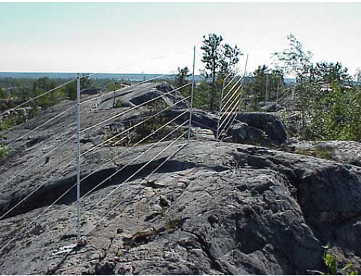
This installation involved blasting holes into the rock to insert the fence posts.
